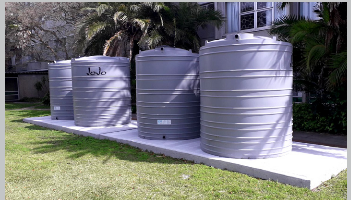
Water storage tanks (48 x 5000L) and related reticulation and pumps for residences on South Campus
