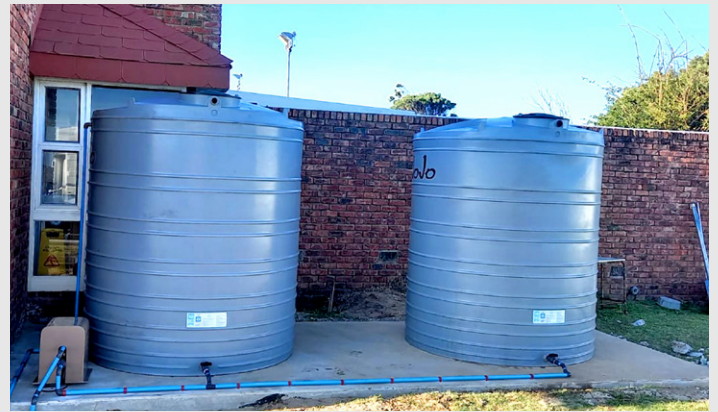
Water storage (26 x 5000L) for critical buildings on North and South Campus (Covid Clinic included)
