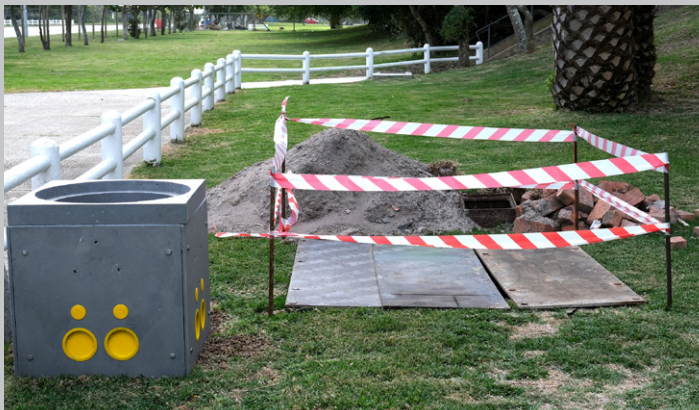
Installation of new water meters on South Campus and remote water reading devices linked to our Building Management System (BMS)
