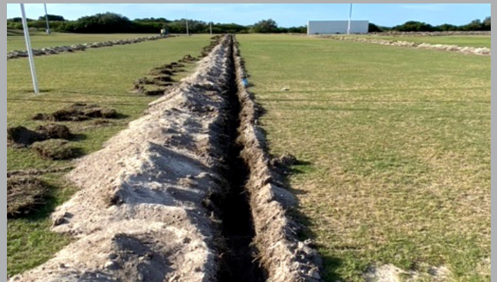
The Return Effluent (RE) Scheme: Installation of 3 new irrigation systems on the Cricket C and Rugby B fields on South Campus
