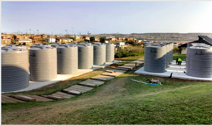
Provision of water storage (20 x 5000L) and related pumps and reticulation for Missionvale Campus
