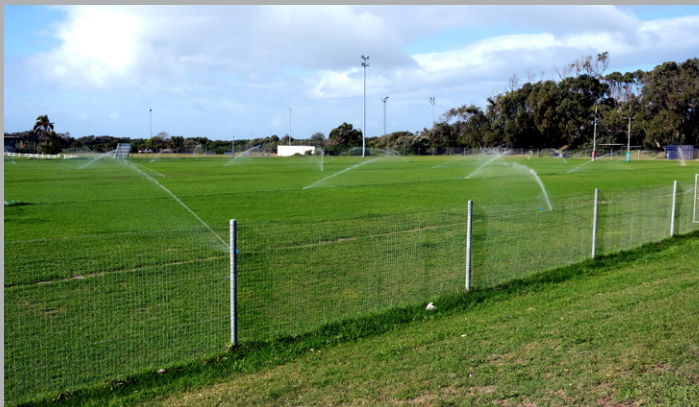
The Return Effluent (RE) Scheme: Installation of 3 new irrigation systems on the Cricket C and Rugby B fields on South Campus
