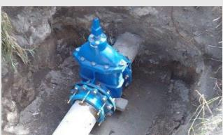
Two 250 millimetre valves have been installed on the South Campus main water system. This provides the ability to manage the campus with greater efficiency during unexpected events such as experiencing burst pipes, or when there is a need to manage alternative sources on campus.
