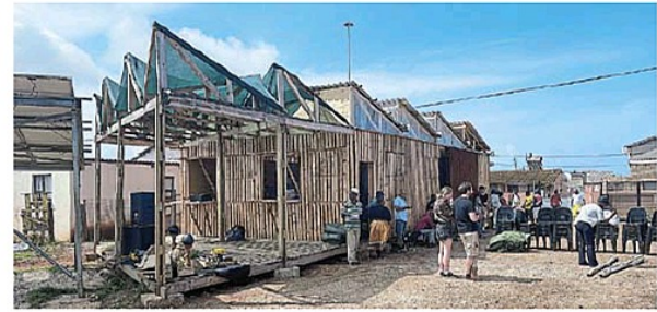
NOW THAT'S CLEVER: The smart building made of recycled pallets Picture: DANIEL HULSEWEG
